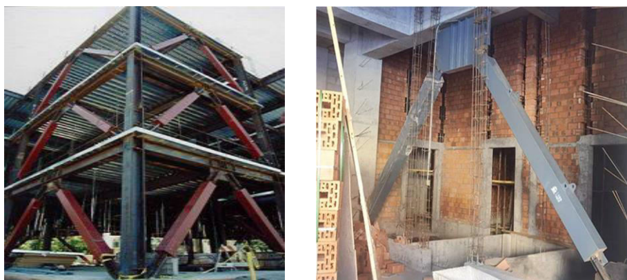
Figure 2: Images of Buckling-Restrained Braces
